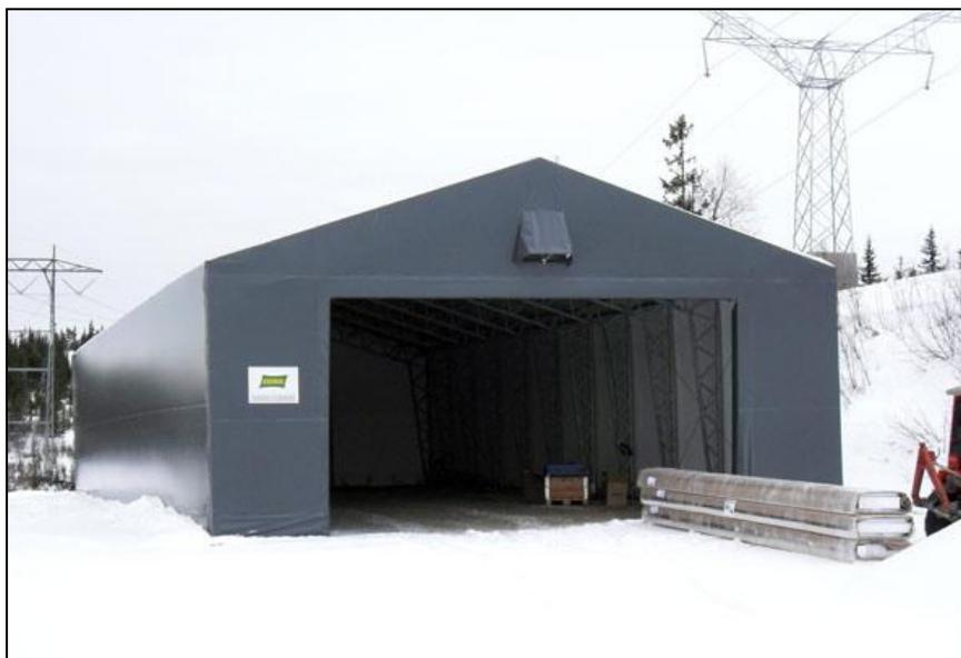
*B: Type of insulated PVC tent which could be used for two-sheet portable curling rink*
