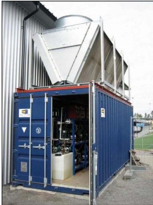
*E: Cooling plans inside a container with condenser fans on top*
